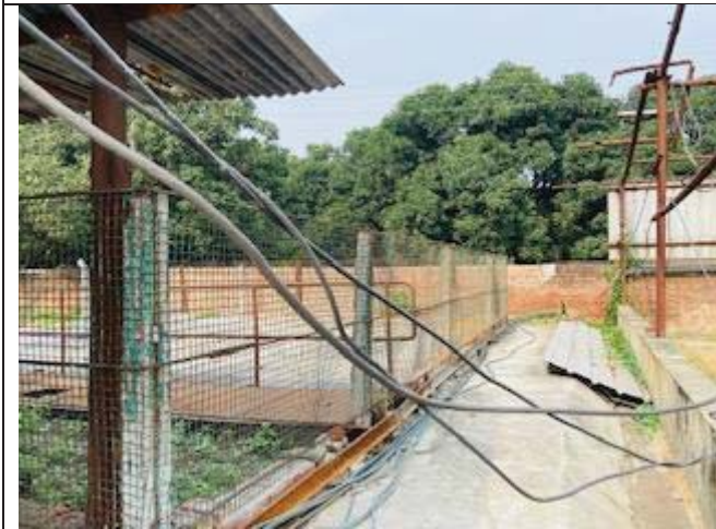
Fig 13: Freshwater line to ETP dismantled
