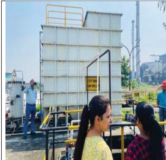
Pic: 9 Sewage Treatment plant
