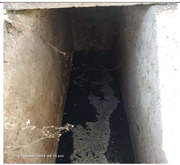
Fig 12: Connecting line with old pumping station blocked
