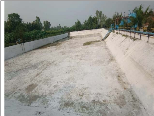
Pic :3 Lagoon for storage of ETP treated effluent
