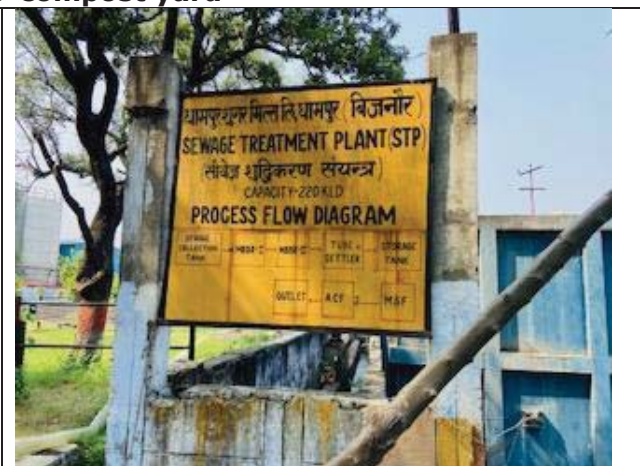
Pic: 5 Sewage Treatment Plant
