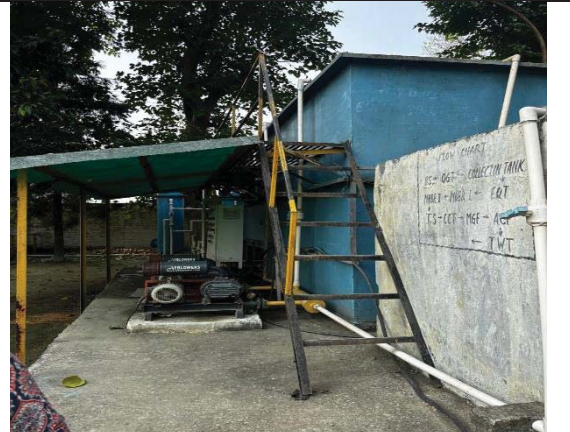
Pic 6: Sewage Treatment Plant
