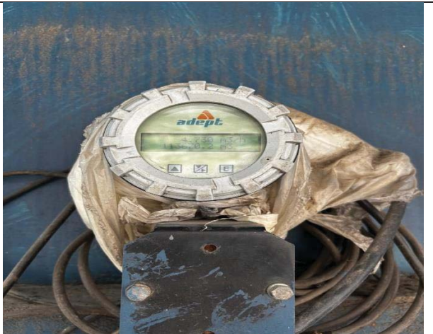
Fig 14: STP inlet flowmeter
