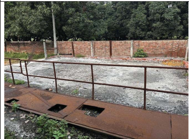
Fig 3: Dismantled old pumping station
