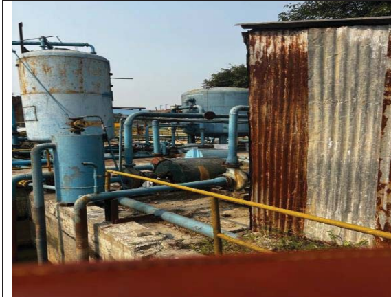
Pic 5: Dismantled the pumping arrangement
